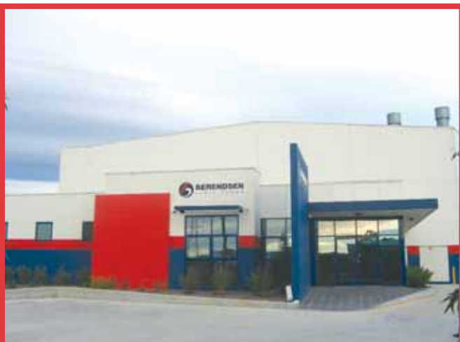
Wetherill Park Branch, NSW
