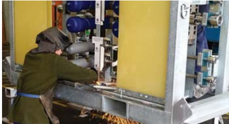
Fabrication and welding of the filtration system taking place at our Newcastle brach by qualified weld staff.
